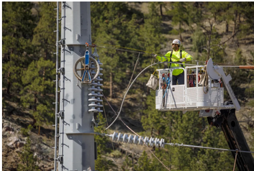
Powering Estes Park, Transmission Line Rebuild Completed October 2023 | Estes-Flatiron, Colorado
