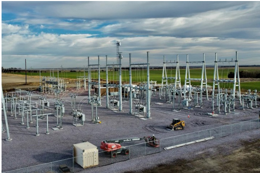
Chamberlain Substation Construction Utility Services Chamberlain, South Dakota
