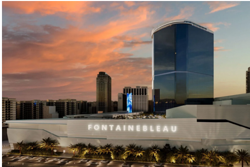
Fontainebleau Remodel Electrical, Mechanical, and Fire Protection Services Completed December 2023 | Las Vegas, Nevada
