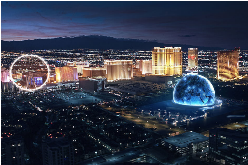
MSG Sphere Construction Electrical, Fire Protection, and Utility Services Las Vegas, Nevada
